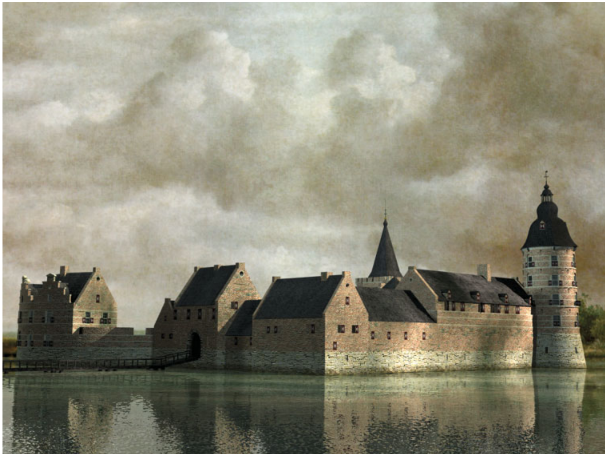
Figure 4. Stevensweert Castle, sixteenth century, DeroDe3D, 2000.
